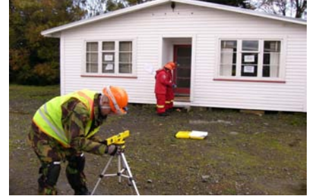
Above: Improvised structural monitoring using laser level on Rescue Command Tactics course.
